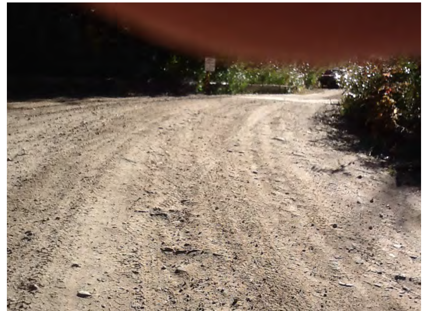
Right approach facing structure
