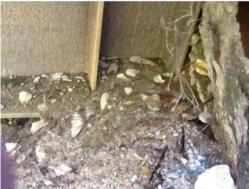
Left Bank Abutment when facing downstream
