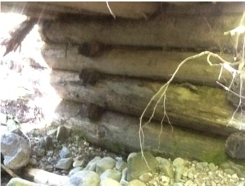
Right Bank Abutment when facing downstream
