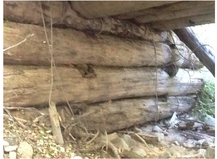
Left Bank Abutment when facing downstream
